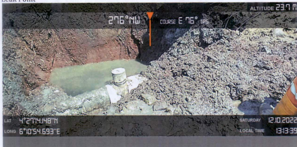
Repaired Point Primed
